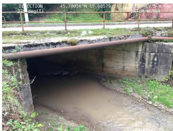
Slika 1.3-7. Most na stac 2+909,0
